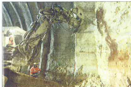
Photo 13. Excavation bench in progress.
