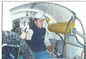
Telescopic thrust station
